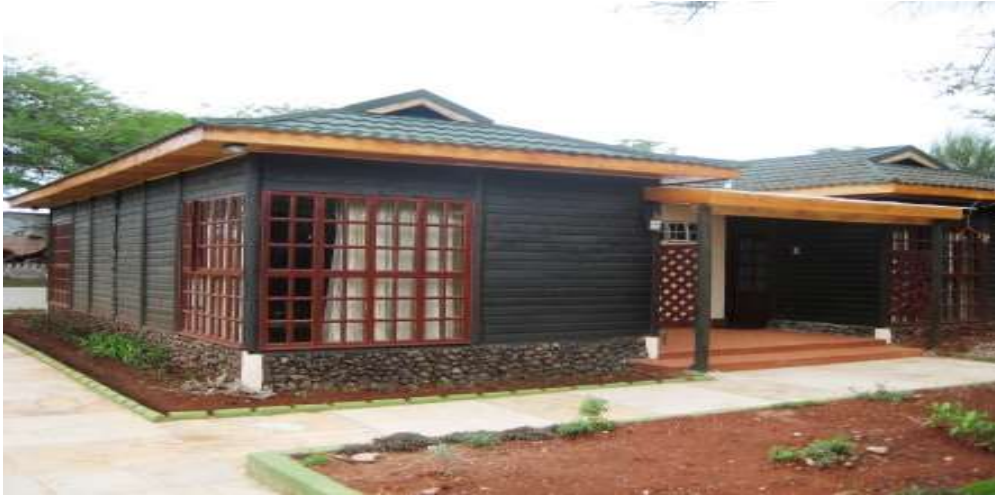
Plate 2.7: Pre-Fabricated Timber Housing
