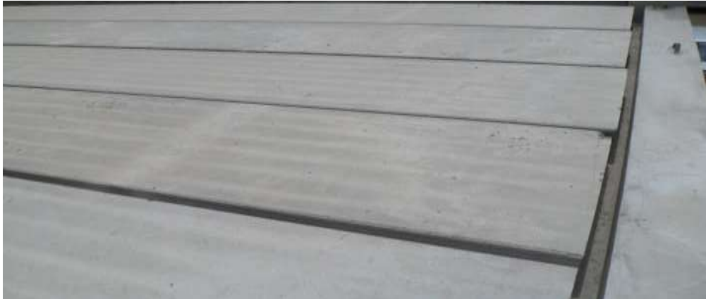
Plate 2.5: Precast Concrete Panels
