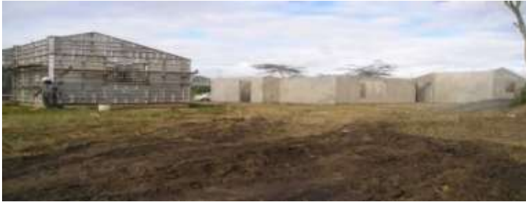
Plate 2.10: Monolithic Construction Using Preconfigured Formwork
