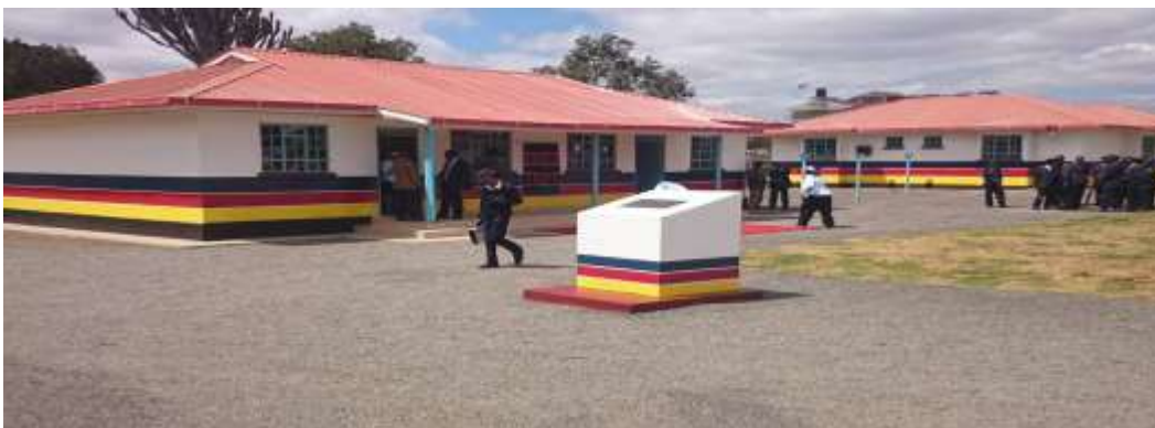
Plate 2.3: Police Housing at Nyeri Showground Made from EPS
