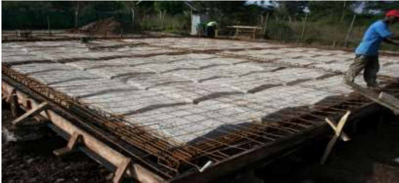
Plate 2.9: Waffles for Suspended Floors
