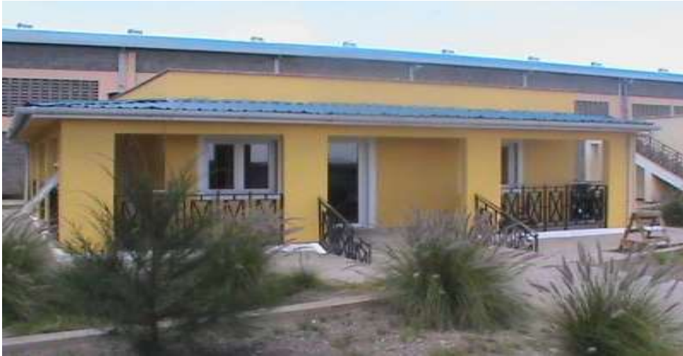
Plate 2.2: EPS demonstration unit
