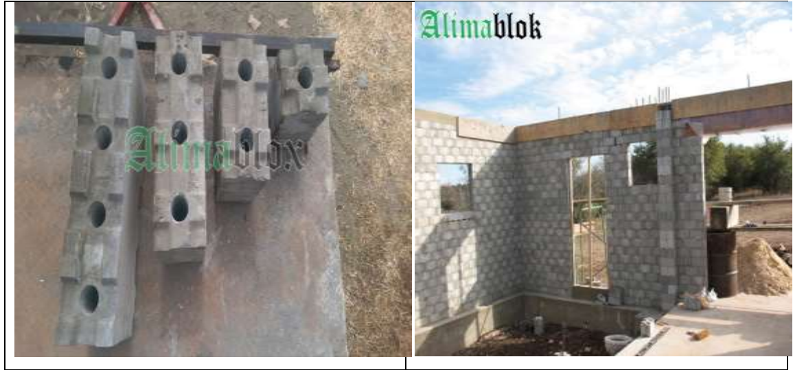
Plate 2.6: Blocks and Demonstration Unit Made from ICB
