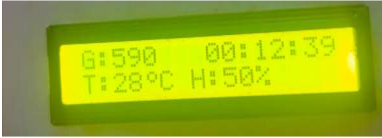
Plate 3.4: The LCD display when the system under normal conditions of temperature and gas concentration.
