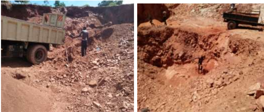
Plate 4.1: Manual loading of Murrum Plate 4.2: Manual loading of Sand
