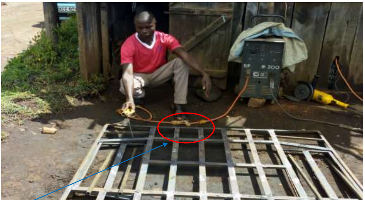
Photo 4: Worn out insulation on an electrical cable for arc welding machine.
