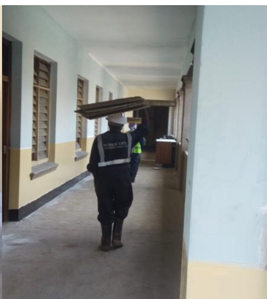
Plate 4.4: Workers carrying heavy materials
