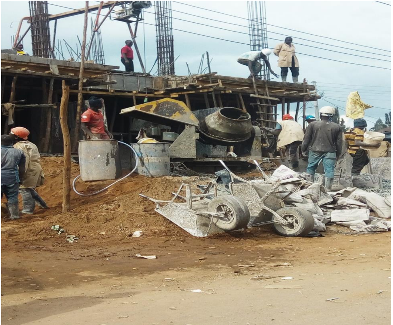
Plate 4.5 Typical construction site
