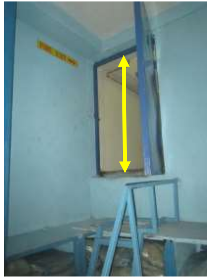
Plate 4.6: Emergency exit access with a height of 76 centimeters
