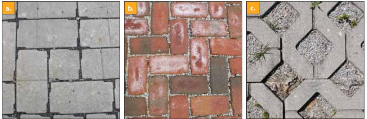
Plate 2-2: (a) Permeable concrete pavement, (b) Permeable brick pavement, (c) Permeable grid pavement (Agouridis et al., 2011)
