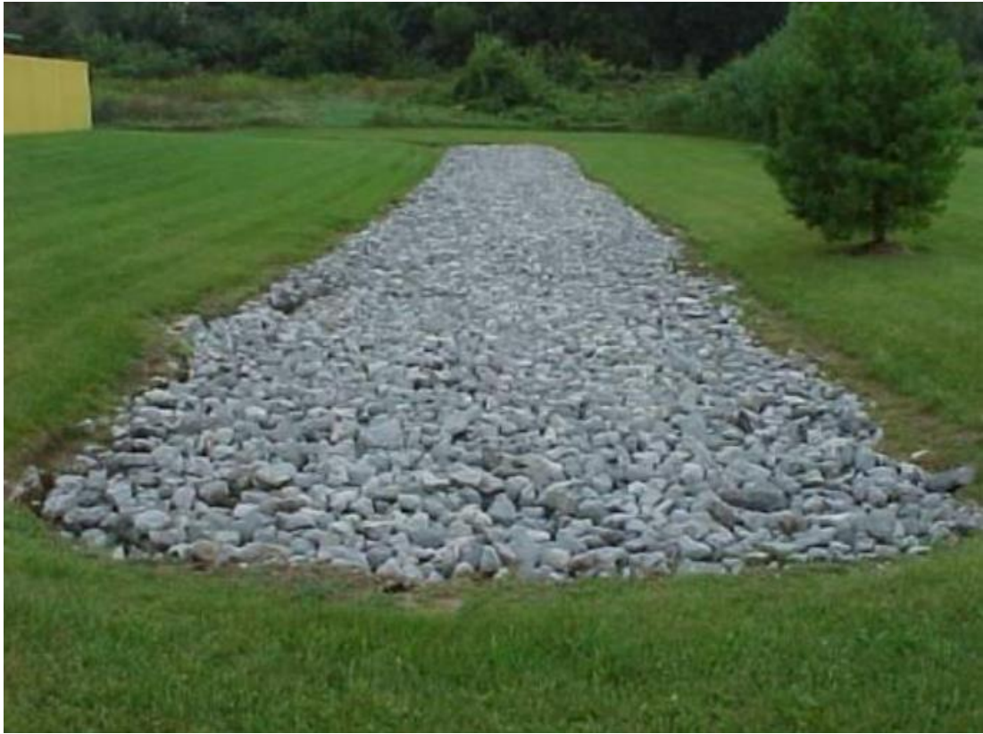
Plate 2-4: Infiltration trench (Rossman, 2016)
