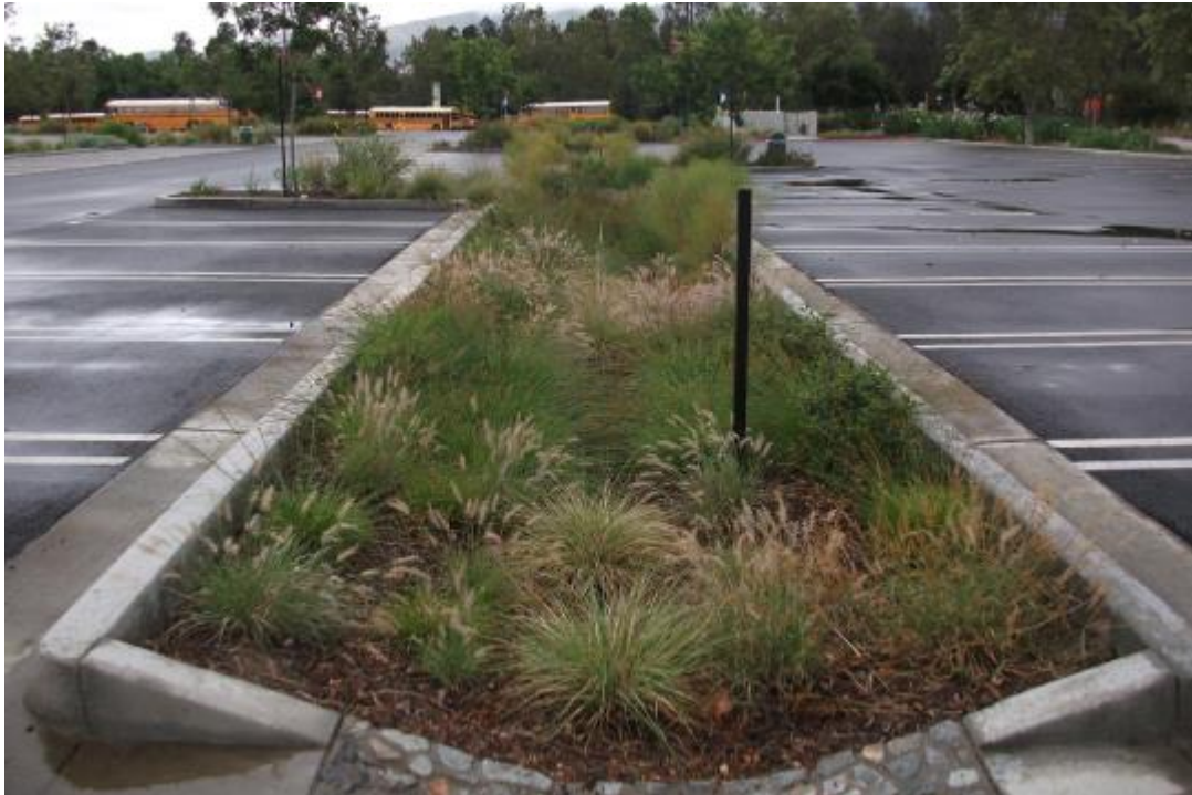
Plate 2-3: Vegetated swales (Singapore National Water Agency, 2018)
