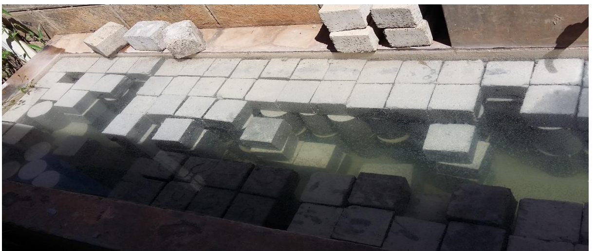
Plate 5: Curing concrete
