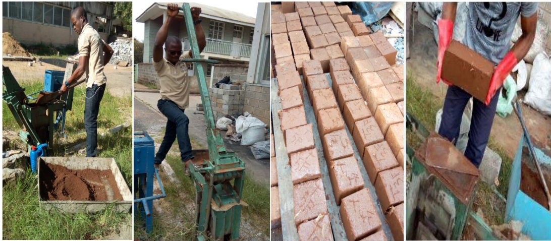
Figure 3.5: Making of compressed stabilized prism and cubical blocks.
