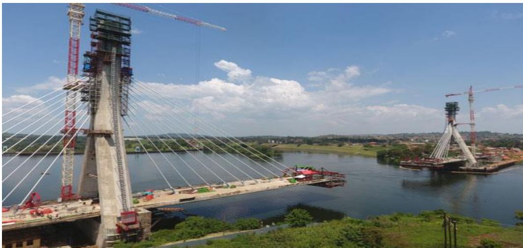
Figure 2-3 Nile River suspension bridge being constructed in Uganda
