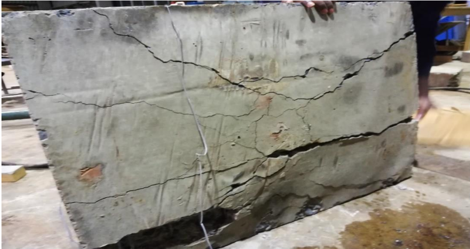
Plate 4-8 Failed Deck Slab – design strength of 30MPa.
