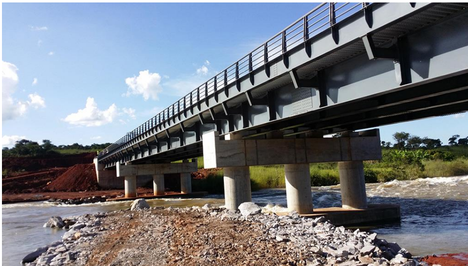
Figure 2-8 Typical composite deck
