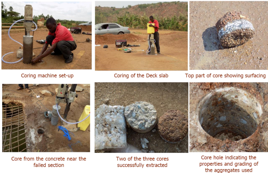
Plate 3-2 Core Testing being done on the deck's slab
