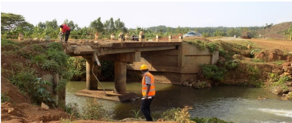
Plate 4-1 Bridge geometry as observed on site
