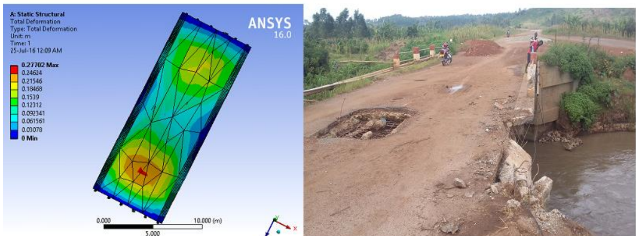
Figure 4-14 Comparison of the Numerical analysis results with the failure of the Manafwa Bridge
