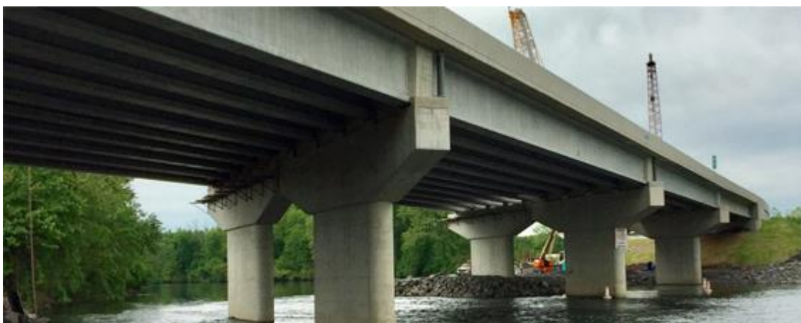
Figure 2-1 Simply supported I-girder bridge structure
