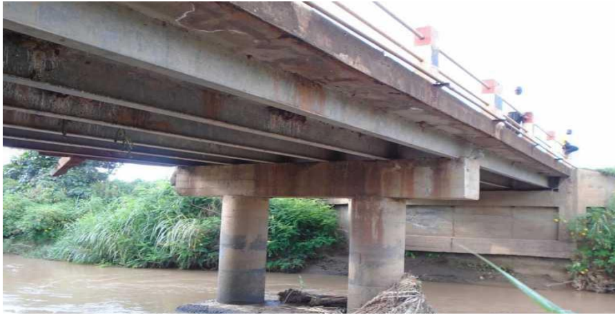
Plate 4-3 Bridge underside showing steel beams and pier.
