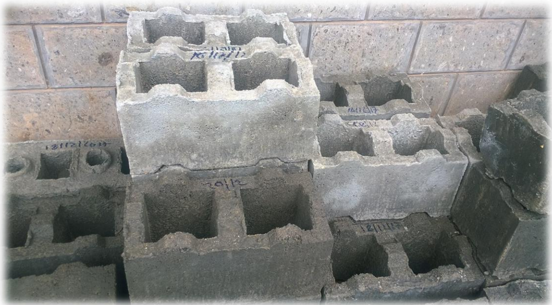
D6: Dry stack hollow sandcrete blocks on curing bay.
