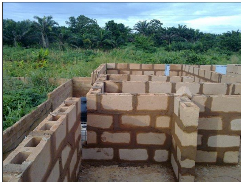
Plate 2.1: Typical Sandcrete wall under construction.
