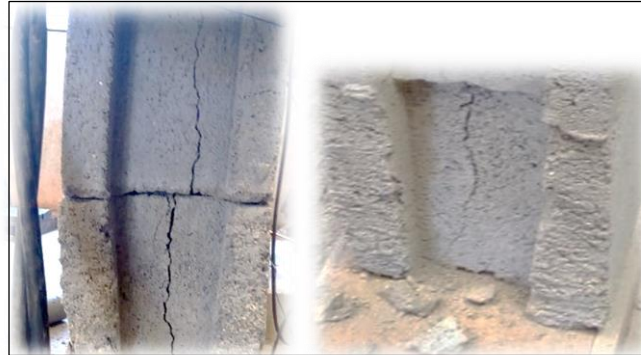
Plate 4.5: Vertical cracks developed at the end face of the specimen.
