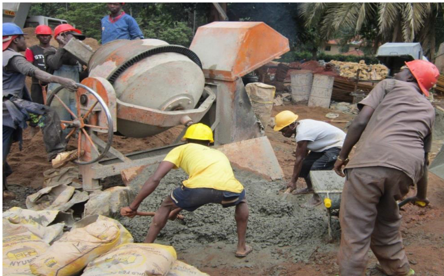
Figure 1.1: Mixing Structural Concrete in Nairobi (Figueroa, 2014).
