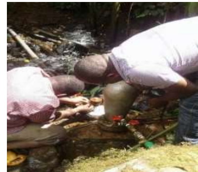
A water hydrum being installed in central Kenya
