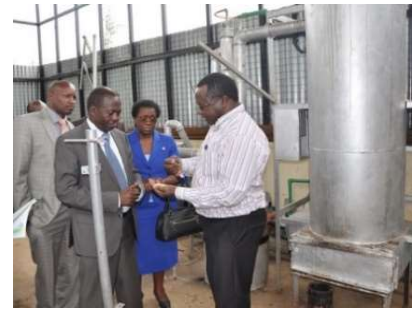
Hon. Cheboi (Govenor Baringo County) following explanations on the working of the gasifier.
