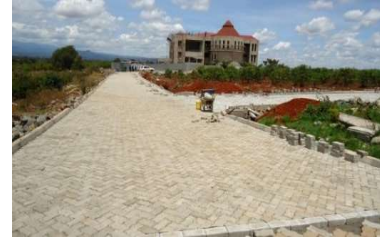
Construction consultancy work by SMARTEC at DKuT
