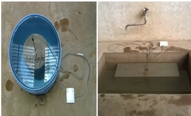
Fig.2. Recording of internal concrete temperature
