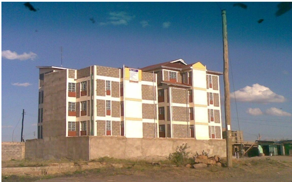
Plate 2: Finishes to a recently completed building in Tassia II, Nairobi.
