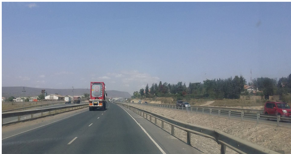
Figure 2 Nairobi to Mombasa road at Athi River
