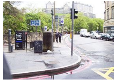
Fig. 8.5: Utility boxes constrains free pedestrian movement, from www.commonswiki.org on 3 Sept. 2010.
