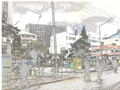
Plate 10.3: Overhead utilities should be undergrounded whenever feasible, by Author, 2010
