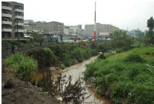
Plate 1.2.9: Dilapidate built fabric and unkempt natural surroundings. (Source: Author, 2007)
