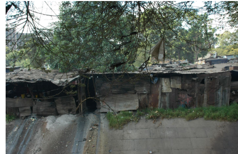
Plate 1.2.11: Informal structures draining waste into the river. (Source: Author, 2007)
