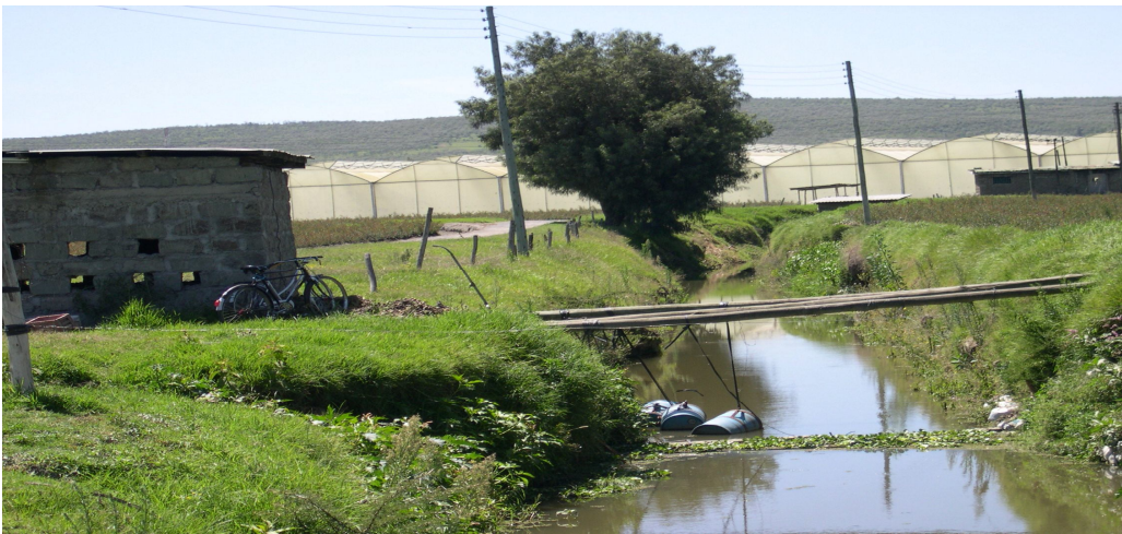
Plate 1.7. Water Abstraction Canal connecting the Lake to a Flower Farm
